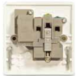
Angled in-line colour coded captive terminals
